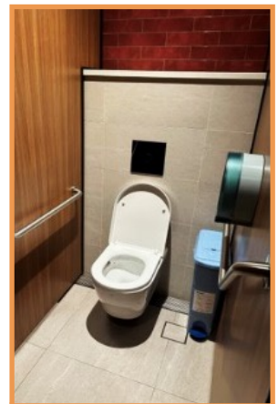
Sanitary bins in female toilet
