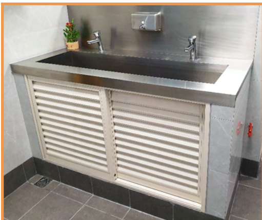
Vanity top-cum-wash hand basins to be provided outside toilets for common use by male and female users
